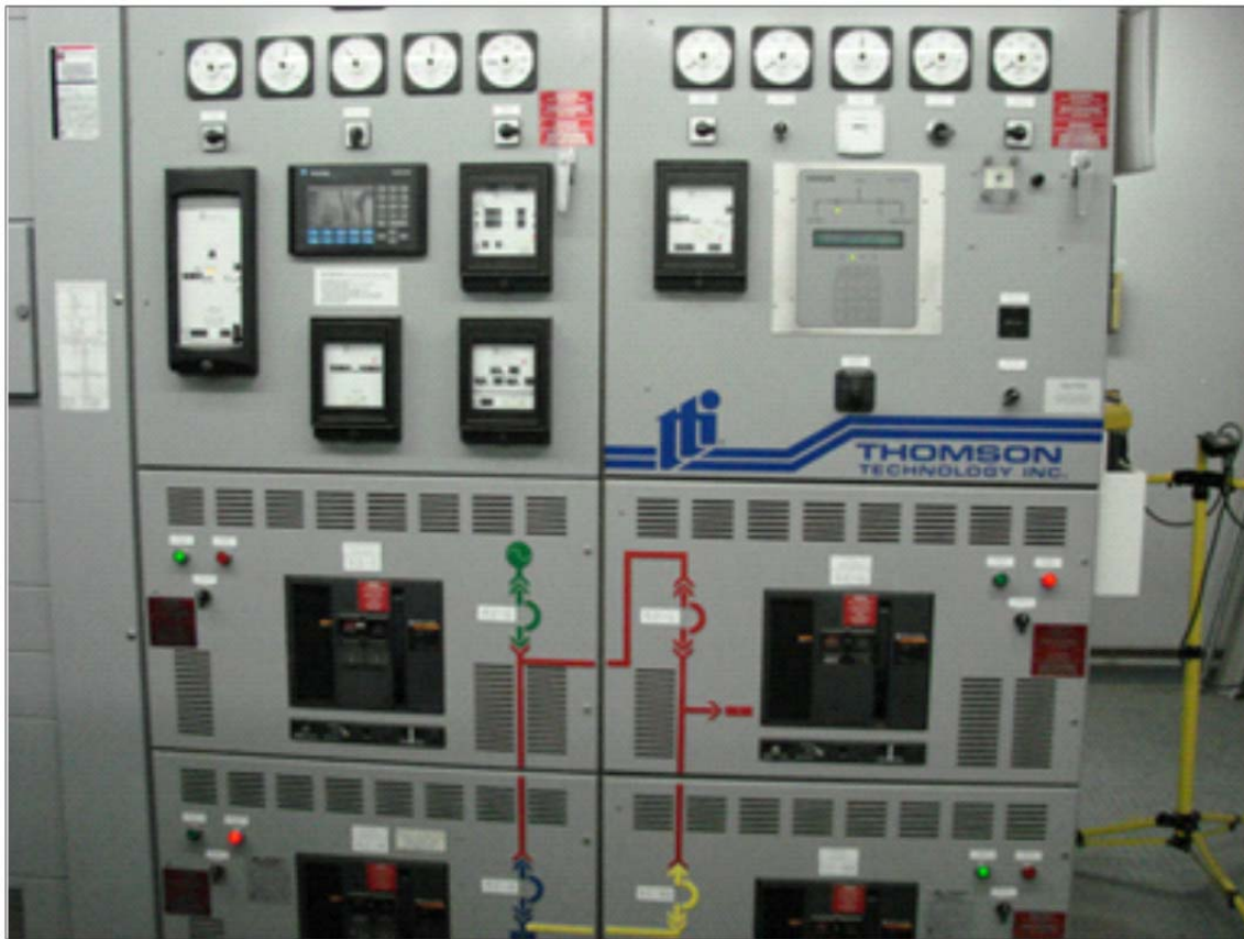
Figure 3-8. Transfer panel (source: Toronto International Airport)
